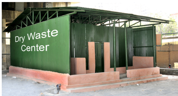
Dry waste collection center
